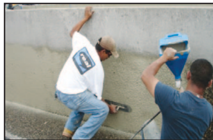
APPLICATION—BY SPRAY / TROWEL
