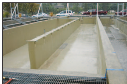
RACEWAY SURFACE COMPLETELY RESTORED
