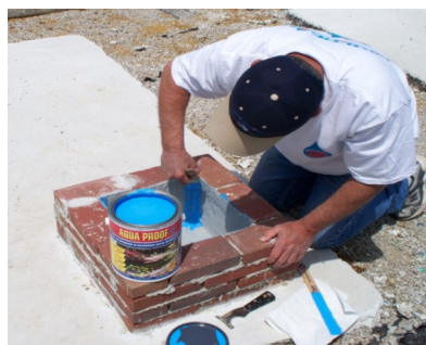
Brush waterproofing membrane into all corners.
