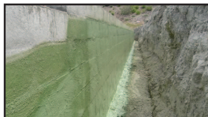
READY FOR BACKFILL
