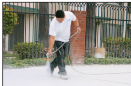
SECOND COAT (FULL STRENGTH COAT) CAN BE APPLIED BY AIRLESS SPRAYER OR ROLLER.
