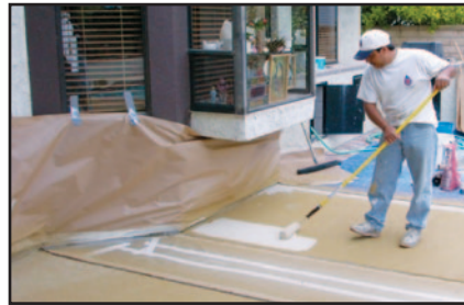
APPLY DILUTED FIRST COAT OF ACRATHANE COLORSEAL WITH ROLLER.
