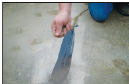
BROADCAST 16-20 SILICA SAND INTO WET SPEED BOND. BRUSH OFF ANY LOOSE SAND WHEN DRY.
