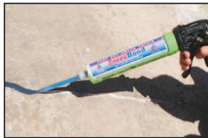
FILL CRACK WITH SPEED BOND
