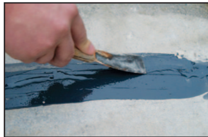
PRESS INTO CRACK AND SPREAD ONTO ADJACENT SURFACE.
