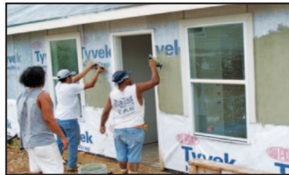
APPLY STUCCO BASE COAT
