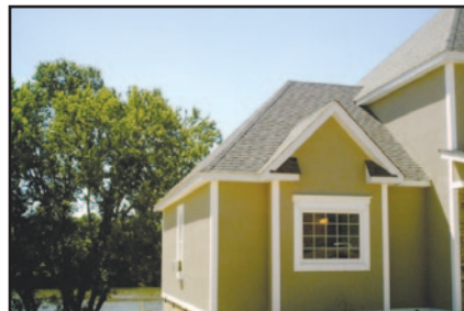
COMPLETED STUCCO PROJECT
