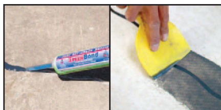
CRACK REPAIR WITH SPEED BOND (SEE CRACK REPAIR SYSTEM).
