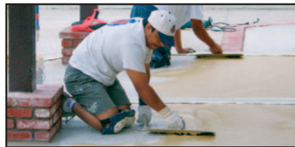
BASE COAT APPLICATION – TROWELED
