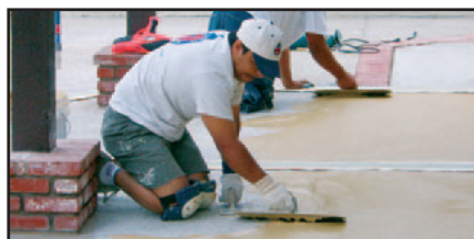
BASE COAT APPLICATION – TROWELED
