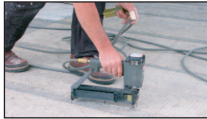
STAPLE METAL LATHE TO DECK
