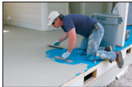
KRETE KOTE/TOP COAT BEING APPLIED
