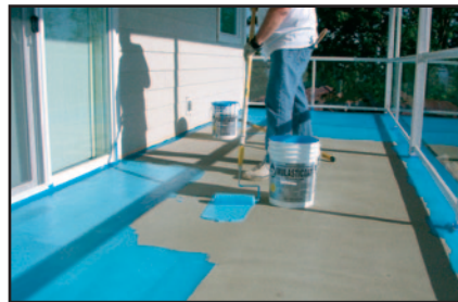
MULASTICOAT® BEING APPLIED (TWO COATS)
