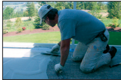
MULTI-BASE APPLIED, COVERING METAL LATHE
