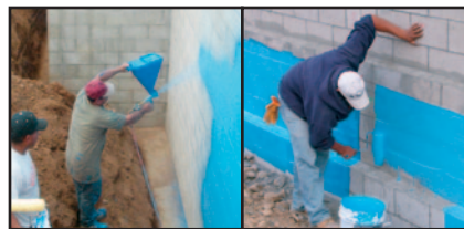
SPRAY APPLIED ROLLER APPLIED
