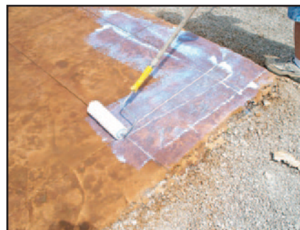
AS SOON AS MULTI-STAIN HAS DRIED, USUALLY THE NEXT DAY, APPLY 2 COATS OF MULTICOAT'S CLEAR SEAL TO LOCK IN THE COLOR AND PROTECT THE SURFACE.
