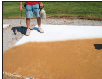
APPLY MULTI-STAIN WITH A PUMP SPRAYER AS SHOWN ABOVE. CAN ALSO BE SPONGED OR BROOMED.
