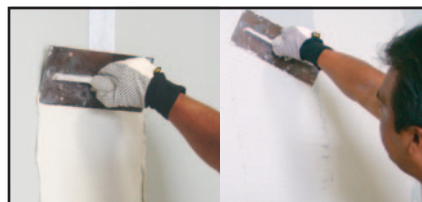
APPLY SMOOTH TO CORNERS AND JOINTS. THEN APPLY STUCCO MIX TO DESIRED TEXTURE
