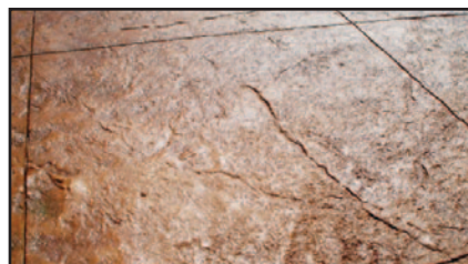
FINISHED OVERLAY STAMP SURFACE.
