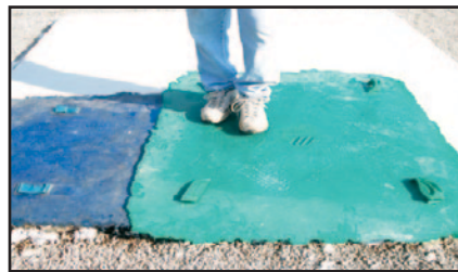
PLACE STAMPS INTO POSITION, MOVING AROUND THE AREA AS NEEDED.
