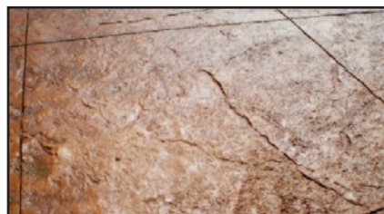
FINISHED OVERLAY STAMP SURFACE.
