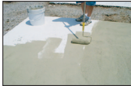
APPLY BASE COAT OF SCRATCH KOTE 2000 AS A BONDING AGENT.
