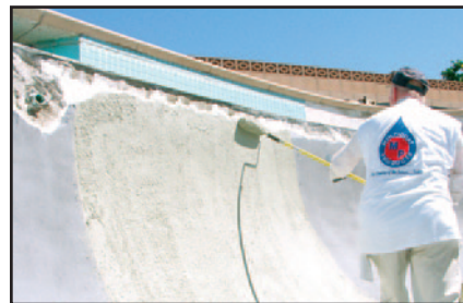
APPLY SCRATCH KOTE WITH NAP ROLLER
