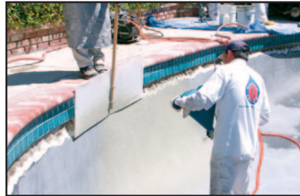
OR APPLY WITH SPRAYER
