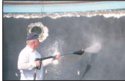
PROPERLY PREPARE SUBSTRATE.
