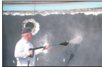
PROPERLY PREPARE SUBSTRATE.
