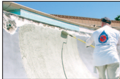
APPLY SCRATCH KOTE WITH NAP ROLLER
