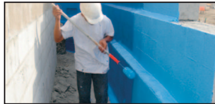
SECOND COAT - MULASTICOAT - ROLLED OR SPRAYED
