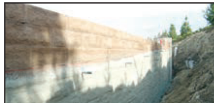
SECOND COAT - MULASTICOAT - ROLLED OR SPRAYED
