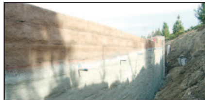
READY FOR BACKFILL
