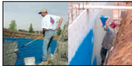
FIRST COAT - MULASTICOAT - ROLLER OR SPRAY APPLIED
