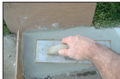
TROWEL OUT LEVEL WITH ADJACENT SURFACE.
