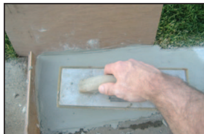
TROWEL OUT LEVEL WITH ADJACENT SURFACE.
