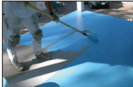
TWO COATS OF "The Blue Stuff" WATERPROOFING MEMBRANE/ MULTICOAT BASE.
