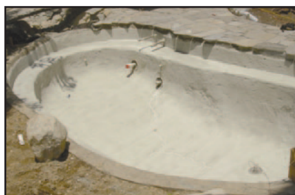
FINAL LAYER OF POND KOTE
