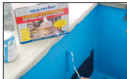
ROLL OR BRUSH COLORCOAT ONTO REST OF AREA MAKING SURE TO COMPLETELY COVER WATERPROOFING MEMBRANE.
