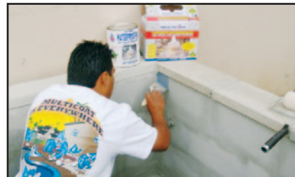
BRUSH WATERPROOFING MEMBRANE INTO ALL CORNERS.
